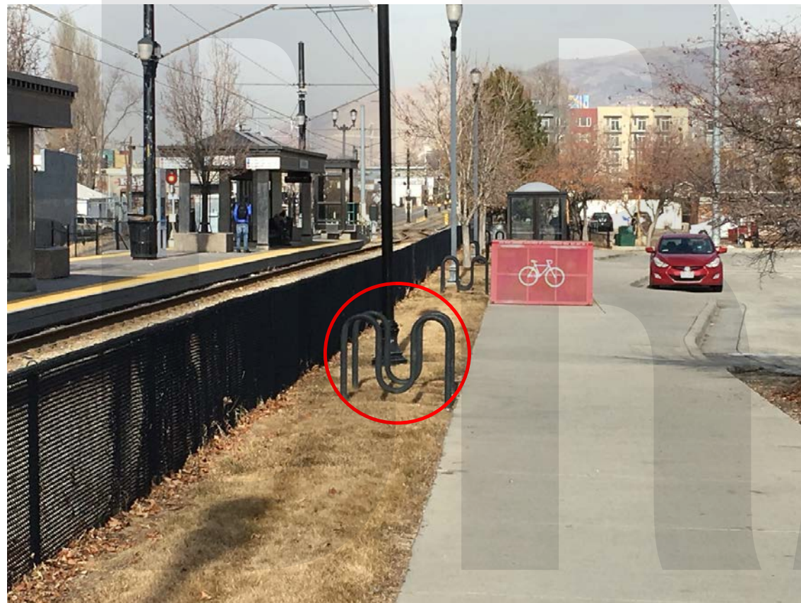
Figure 26 - Improper Bike Racks as Ballpark Station
